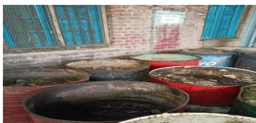
ETP sludge lying undischarged at Loco & Carriage and Wagon Workshop- Dahod at Ratlam Division in WR
